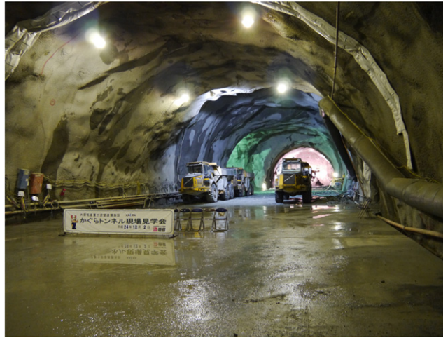
Figure 6. Photograph of the center area. The dimensions are a width of 15 m and a maximum height of 9.5 m.
