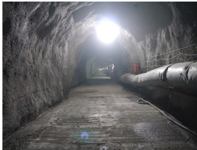
Figure 8. Photograph of the Yarm tunnel. The dimensions of the tunnel are a width of 4 m and a height of 4 m.
