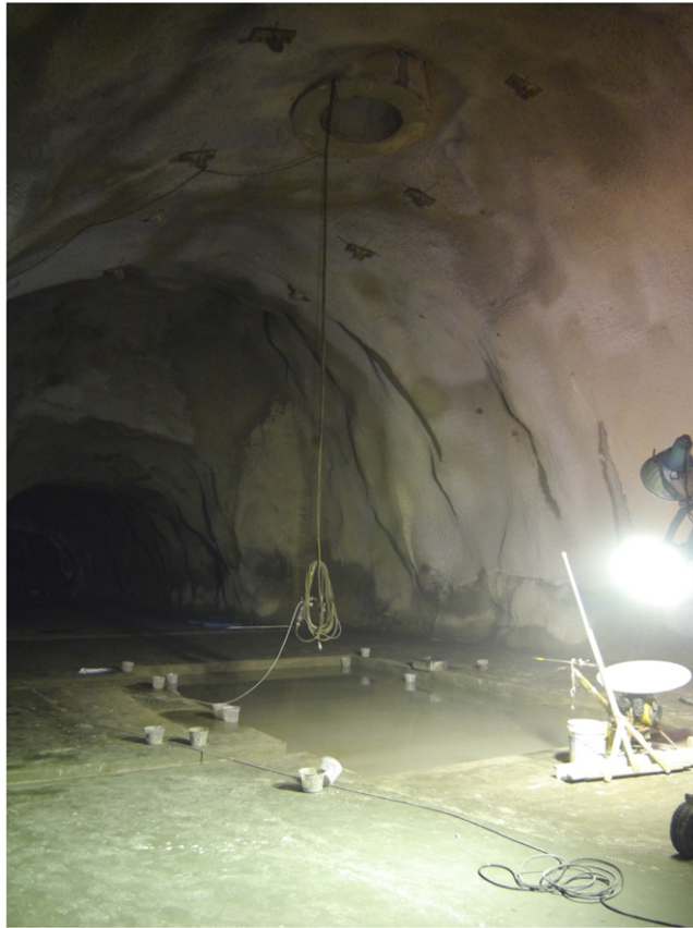
Figure 11. Photograph of the Yend cryogenic mirror room. Included are a pit for a cryostat and a vertical hole.
