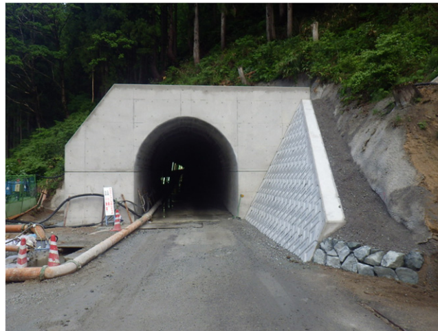
Figure 3. Photograph of the new Atotsu entrance. The dimensions of the entrance are a width of 4 m and a height of 4 m.
