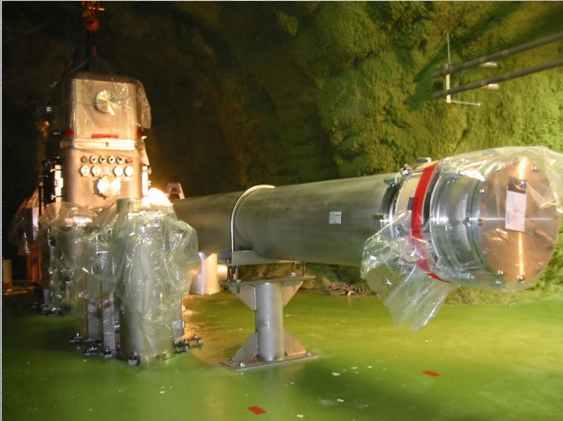
The inline end cryostat has been installed. 2004/09.
